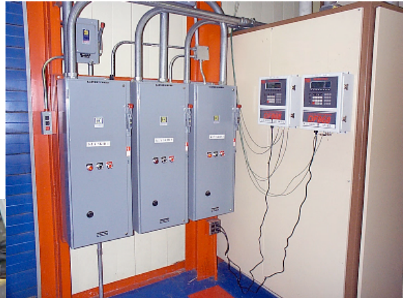
Fig. 6.31 Klystron Motor Panel are monitored are the supply and return pressures and temperatures of the LCW system along with the flow rate of the ICW and LCW.
