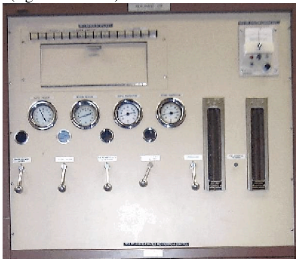
Figure 4.34b, RF Water System Control Panel—Front The supply valve for each circuit is on the front of the cabinet (figure 4.34b), and the return valves are in the rear (figure 4.34d);
