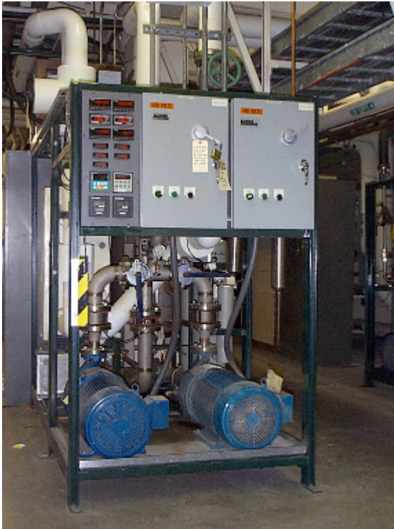
Fig. 6.32 Klystron Distribution Skid
